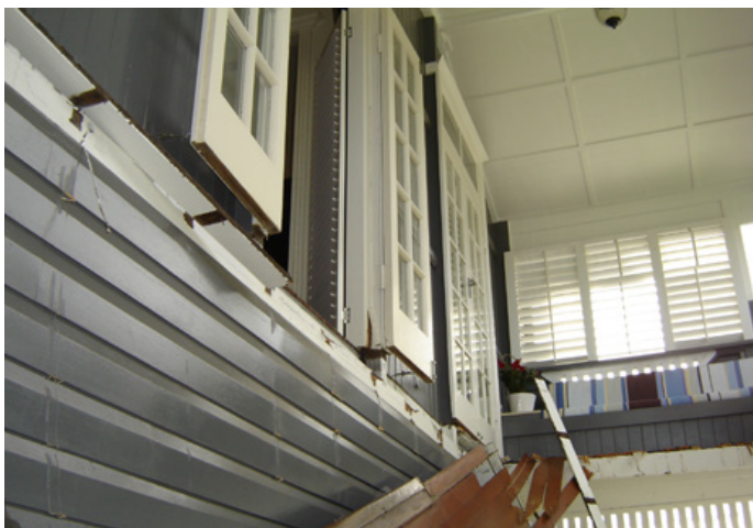
View of internal bearer support at external wall of home
