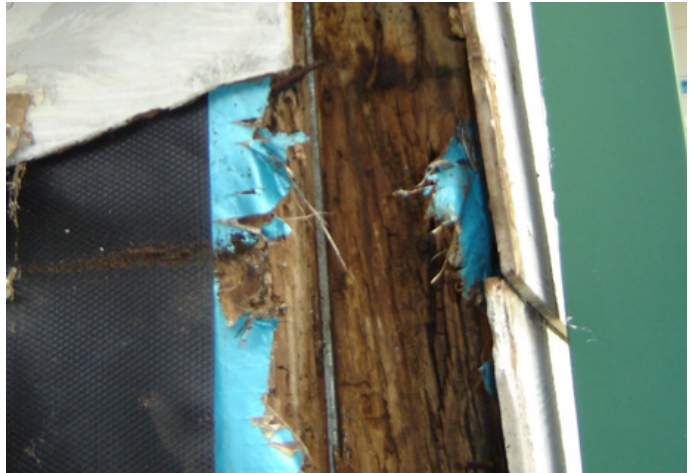
Rotted wall studs below the bearer support joint
